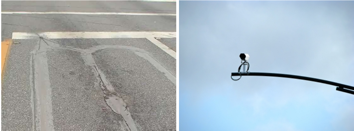
Figure 3.1: An induction loop (left) and traffic camera (right)
