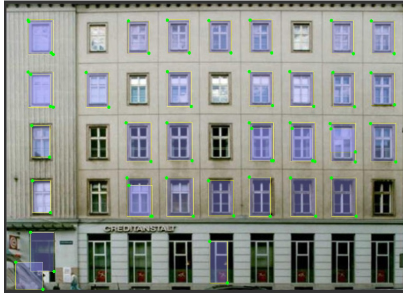
Figure 7: Overlapping window and not all of the window were detected.
