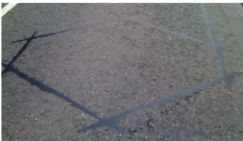
Figure 25 Typical induction loop detector installation
